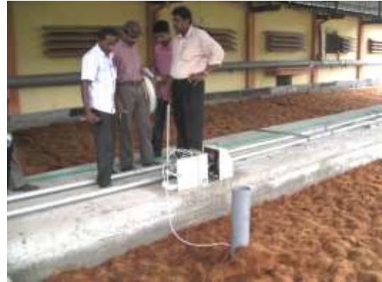
Figure 4. Gas biofilter treating odour from a ossein factory that makes gelatine from animal bones. Sinews separated from bones are rendered to make meat meal pet food. Emissions from meat meal plant is treated in this biofilter.
