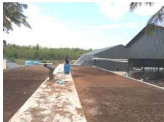
Figure 6. Gas biofilter for odour control in 180 tpd fishmeal plant at Palghat (2014).
