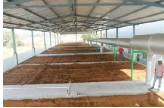
Figure 10 Biofilter for 300 tpd prawn feed factory, Odisha (Licensee: Elixir Enviro Systems Pvt Ltd https://elixirenviro.in/ )
