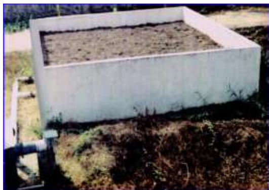
Figure 3. Small Gas biofilter treating odour from tanks of a sewage treatment plant at Cochin International Airport
